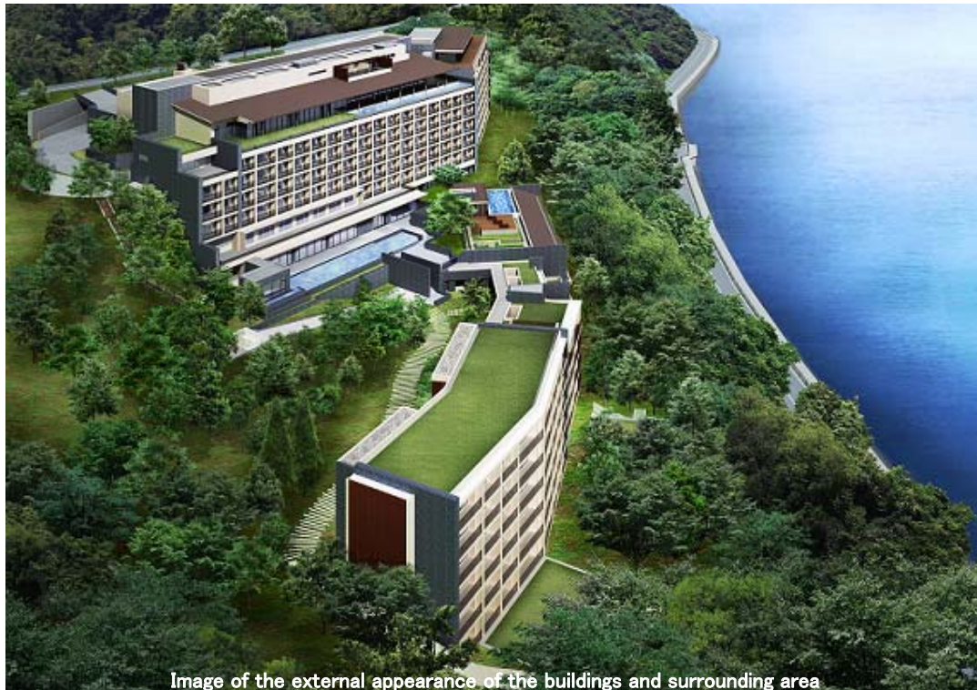
Image of the external appearance of the buildings and surrounding area
