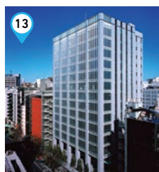
13 Shibuya Minami Tokyu Building
