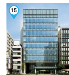
15 Minamiaoyama Tokyu Building
