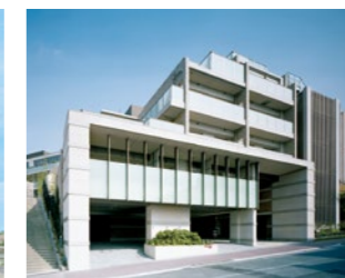
15 Grancreer Fujigaoka Care Residence
