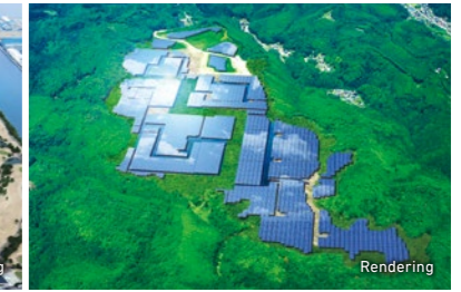
Solar power plant (Nara)
