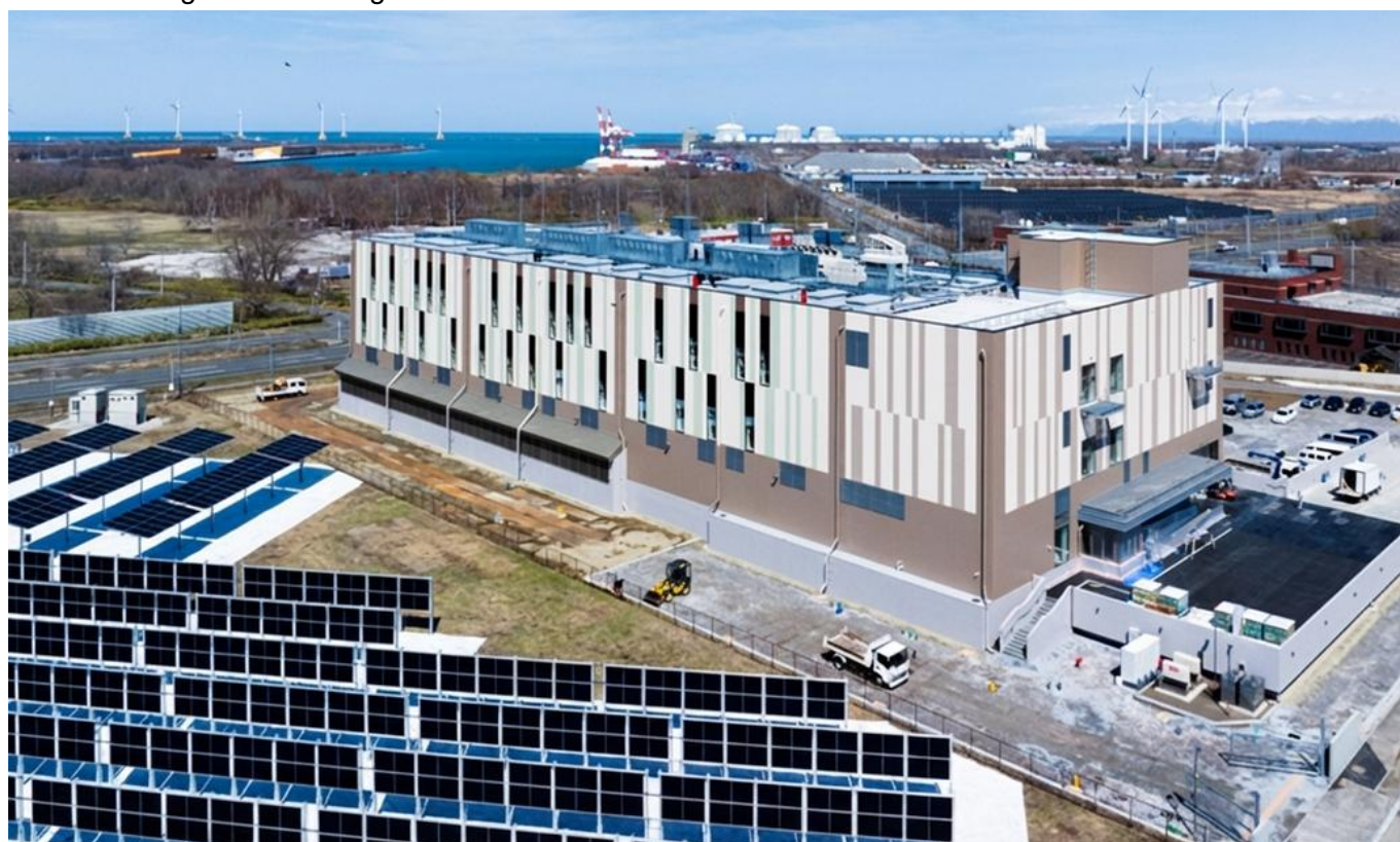
Exterior view of Ishikari Renewable Energy Data Center 1
