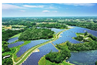
ReENE Namegata Solar Power Plant (Namegata City, Ibaraki)
