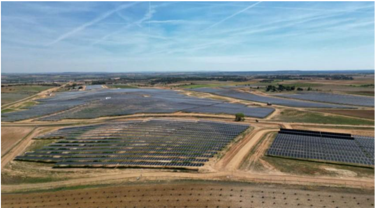
Valdecarretas Solar Power Plant
