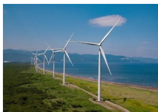
ReENE Zenibako Wind Power Plant (Otaru, Hokkaido)
