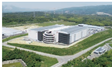
Kuwana Logistics Center
