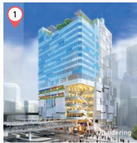
SHIBUYA FUKURAS Completion: October 2019 (planned)
