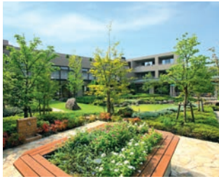
5 Grancreer Azamino Land: Leased* Building: Owned by the operator * Fixed-term leasehold: Until January 31, 2054 (including the period for demolition)
